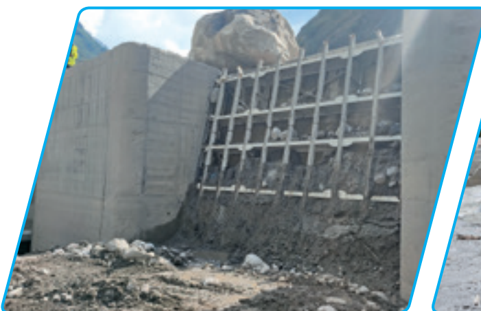
Damages in the intake trash rack
