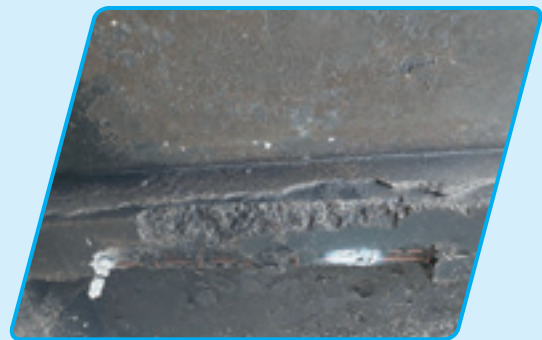
Fire damage observed on the beams of Napi Bibhag building
